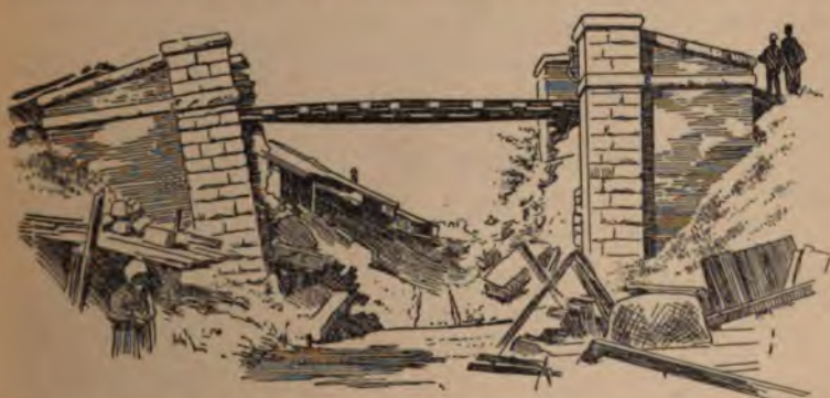
FIG. 65. — The Biwajima railroad bridge in Japan after the earthquake of 1891 (after Milne and Burton).
